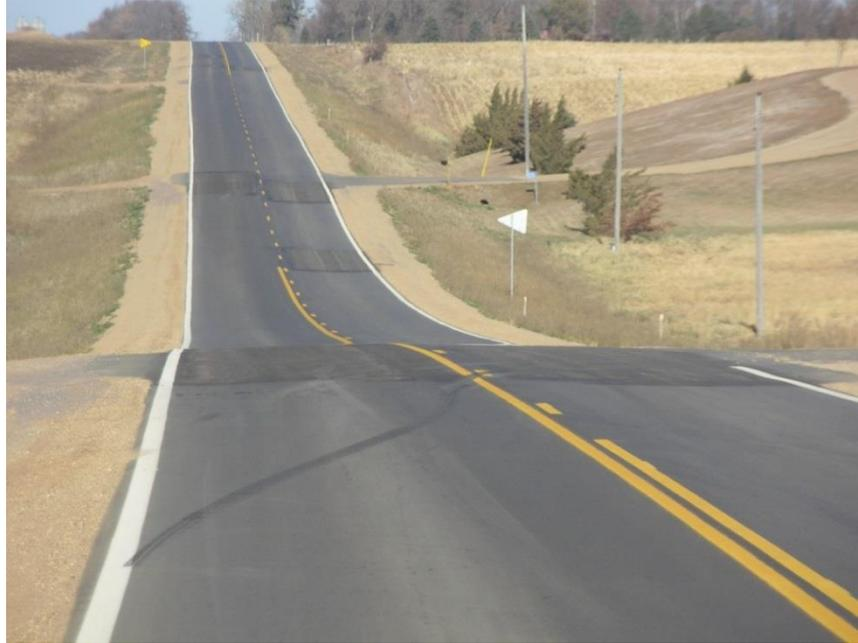
**Figure 600.41** – A recently constructed roadway after surface grinding was completed to improve ride quality.
