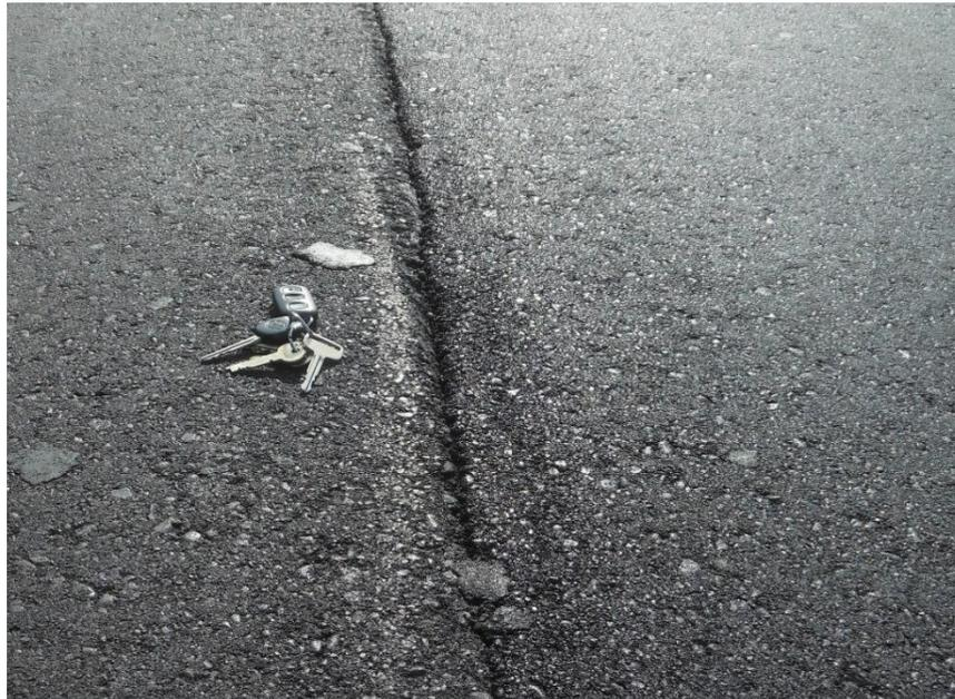
Figure 600.32 – Poorly compacted longitudinal joint
