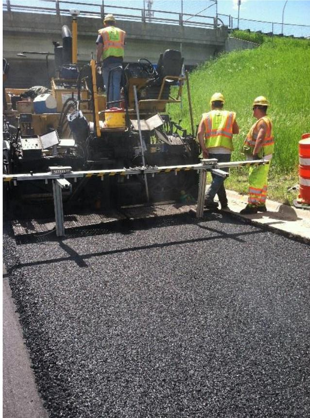
Figure 100.5 – SMA being placed over a bituminous surface.
