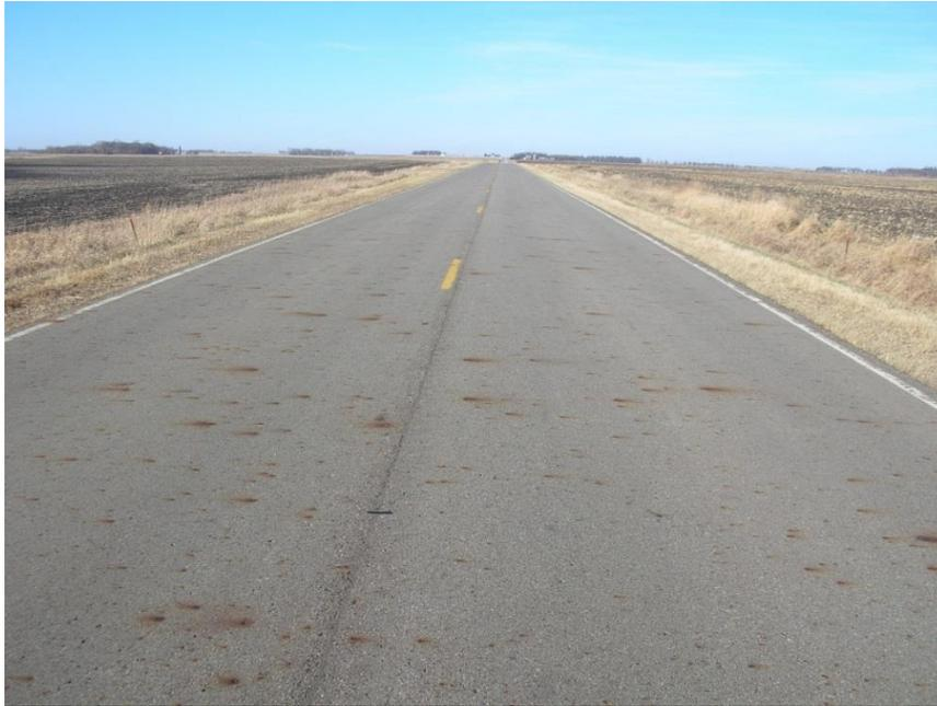
**Figure 600.16** – The effect of excessive Iron Oxide in the bituminous mixture.
