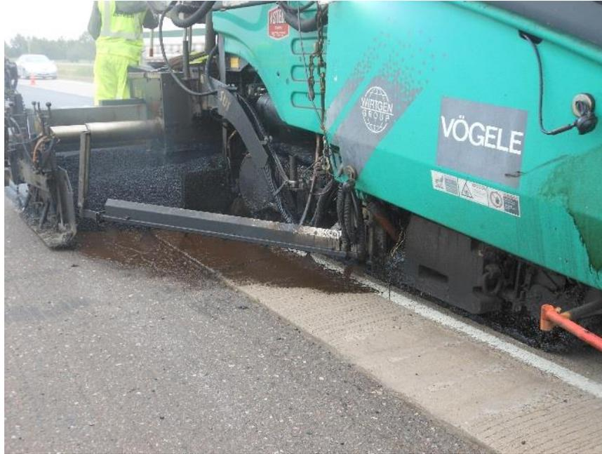
**Figure 100.2** – Spray paver applying tack and UTBWC
