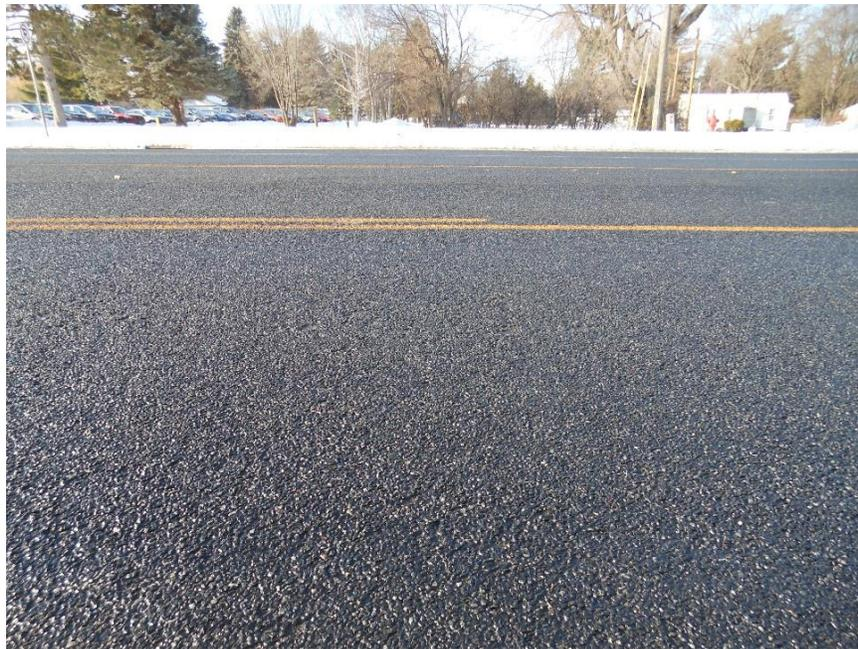
Figure 100.7 – Bituminous Seal Coat
