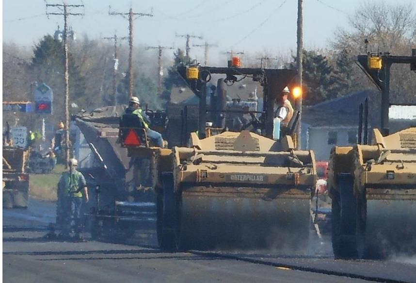
**Figure 500.22** – Compacting an unconfined edge. Note the roller at the front of the train hanging the drum over the edge by several inches.
