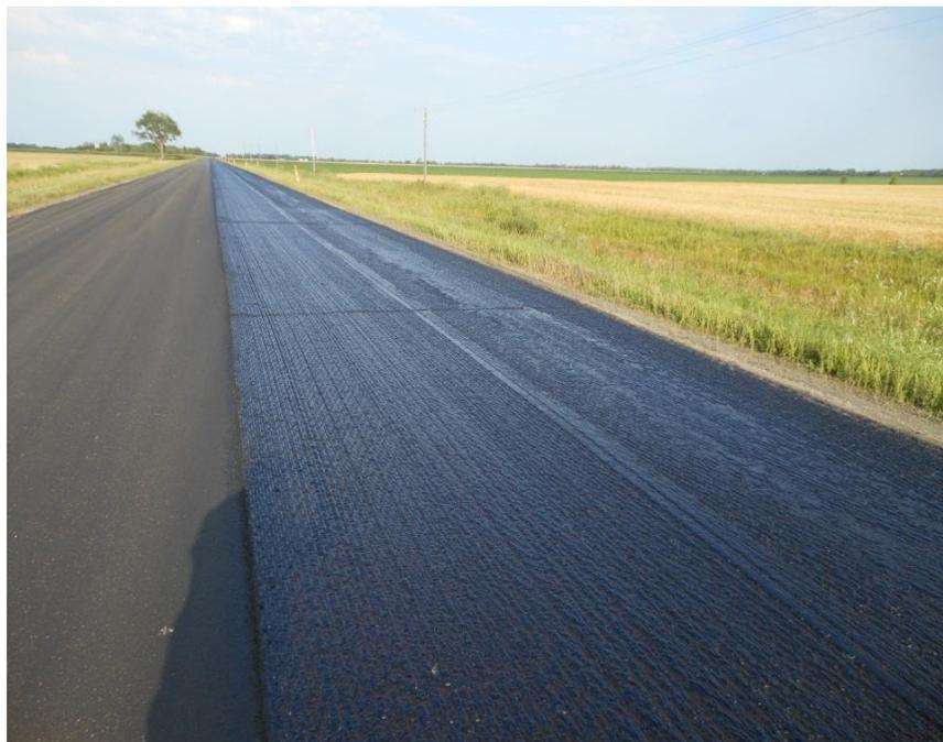
**Figure 100.6** – Bituminous tack coat used to bond an asphalt overlay to the milled surface of an existing bituminous pavement.
