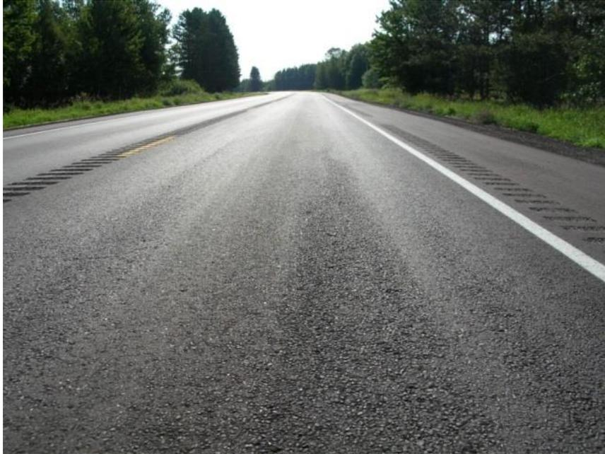
**Figure 600.10** – Severely segregated pavement
