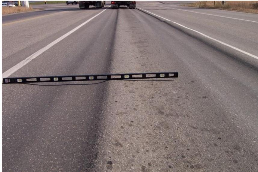
**Figure 100.18** – Pavement Rutting
