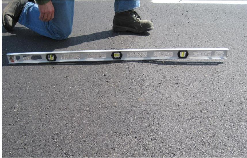
**Figure 600.28** – Bump over concrete joint
