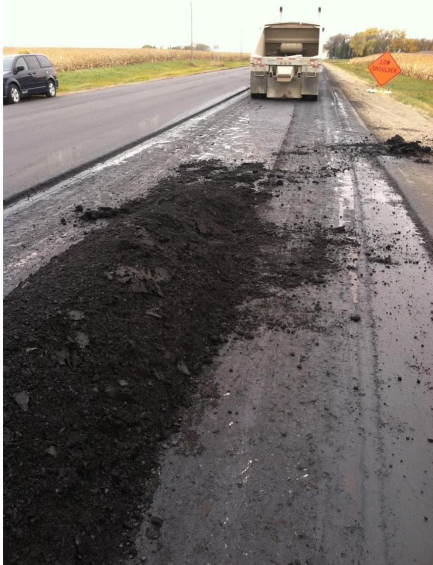
**Figure 600.37** – Chunks of mix in a windrow. These should be removed.
