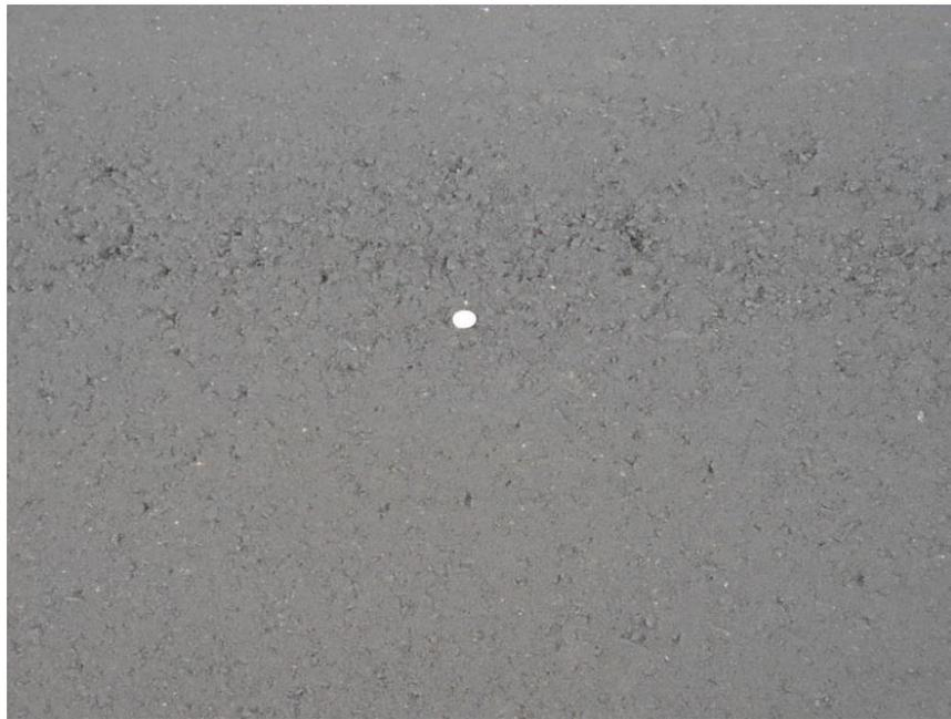
**Figure 600.8** – Slightly segregated pavement
