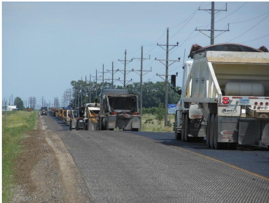
**Figure 600.36** – Excessively long truck queue. The bituminous mixture in the trucks waiting at the far end of the queue will likely have cooled to an unacceptable temperature by the time it gets to the paver.
