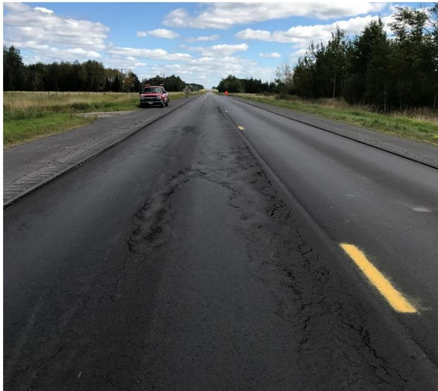
**Figure 600.35** – This is what the road can look like the day after paving in the rain. All of the distressed areas shown will need to be removed and replaced.
