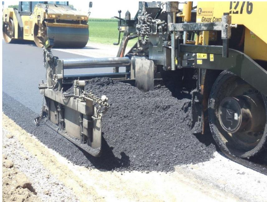
**Figure 600.18** – Excessive material head in front of the screed. The augers should not be buried.
