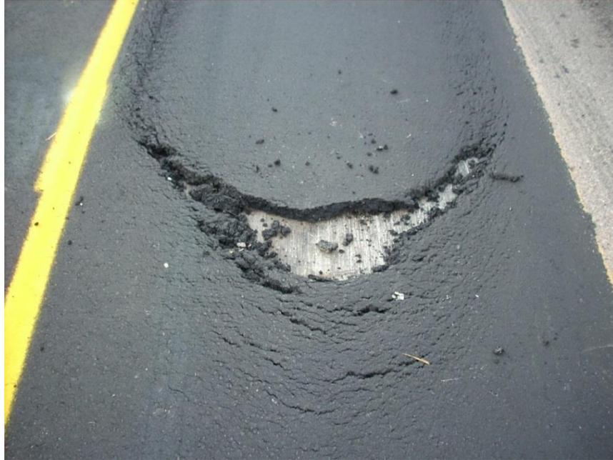
**Figure 600.40** – Longitudinal shoving of the bituminous mat as a result of insufficient or nonexistent tack coat. In this case, the wrong bituminous mixture was used for the application in addition to insufficient tack coat prior to paving.
