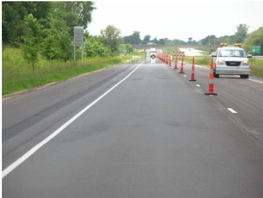
**Figure 600.7** – Chevrons from folding hopper wings
