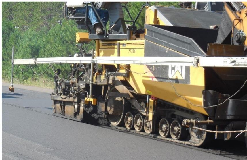
Figure 500.16 – A tracked paver using sonic sensors to adjust the screed.
