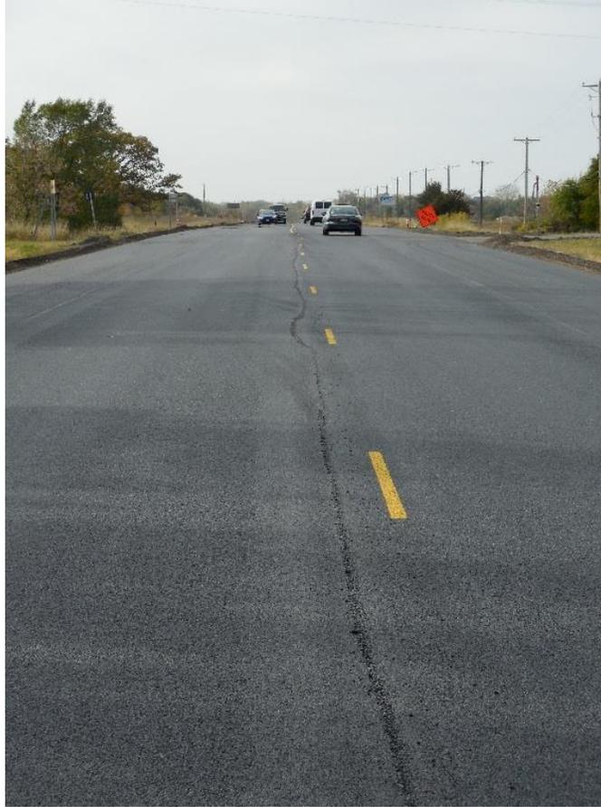
**Figure 600.30** – Wavy Longitudinal Joint
