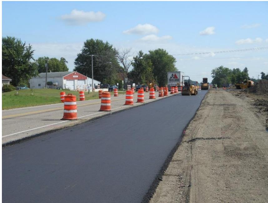
**Figure 500.1** – Paving operation within a traffic control setup.
