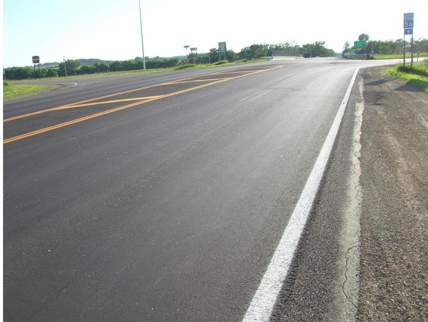
**Figure 100.8** – Micro Surfacing
