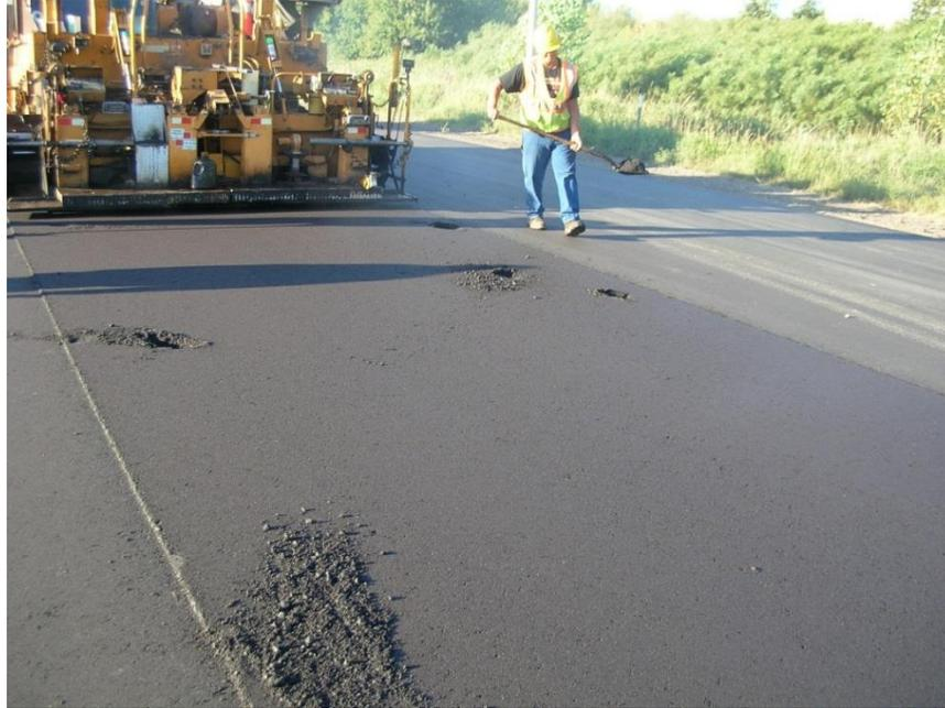
**Figure 600.38** – Removal of chunks from the bituminous mat. The areas will have to be filled in by hand, and will likely be areas of localized segregation. Paving operations should halt if this continues.
