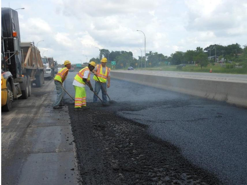
**Figure 600.21** – The result of “paving” without bituminous mixture present in the paver hopper
