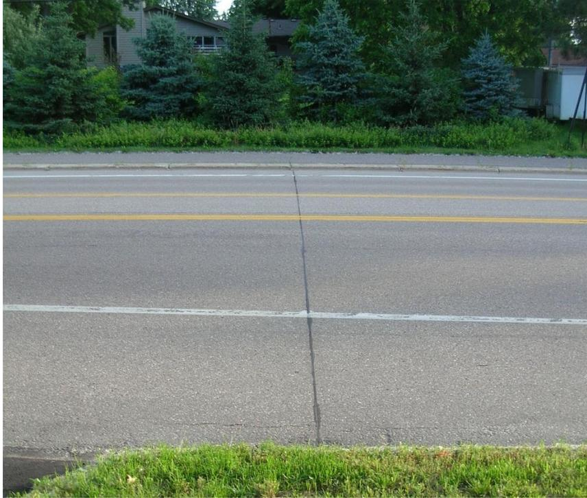
**Figure 200.19** - Saw and Seal roadway
