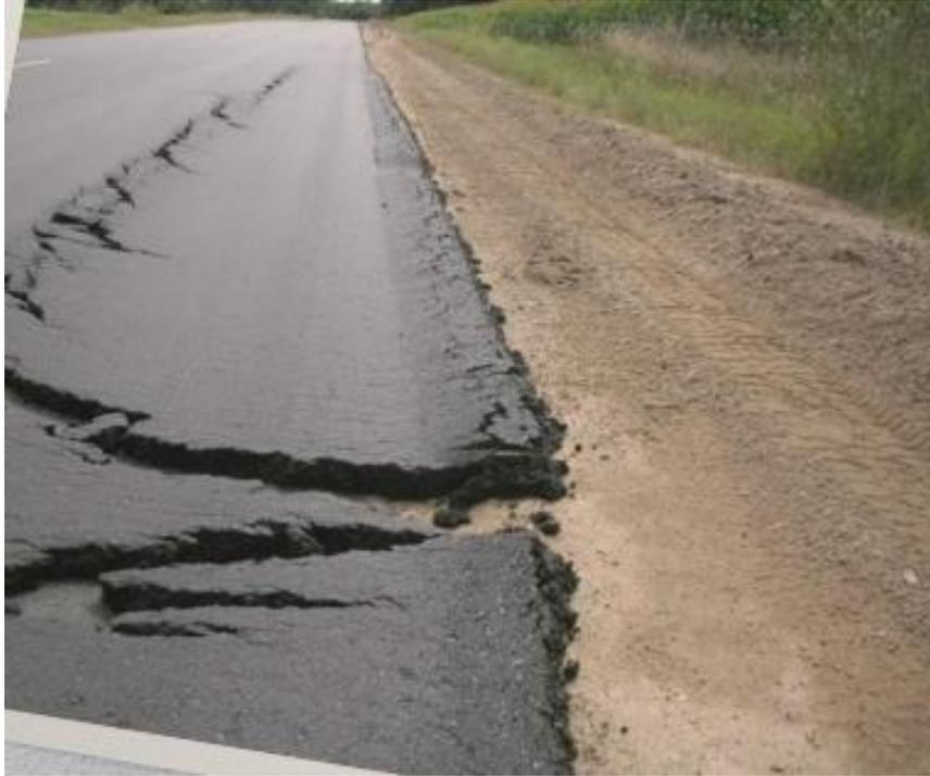
**Figure 600.23** – Yielding of the aggregate base
