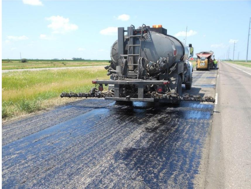
**Figure 500.6** – Tack coat distributor truck. Note the streaked appearance. The Contractor should respray this area to achieve uniform coverage.
