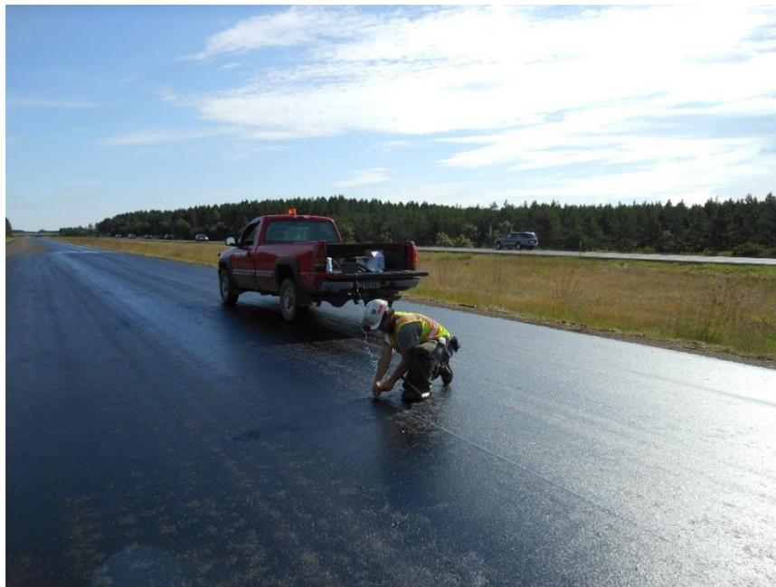
**Figure 600.31** – Contractor setting stringline to guide the paver
