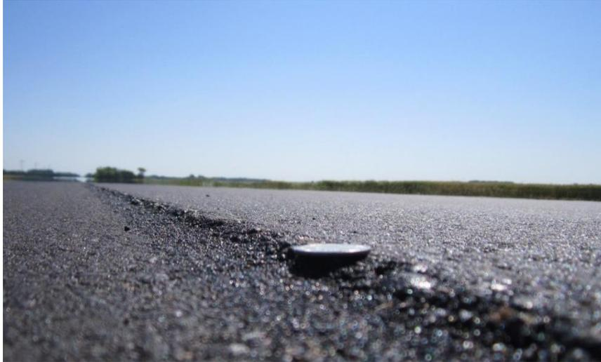
**Figure 600.33** – Excessive height differential at a longitudinal joint
