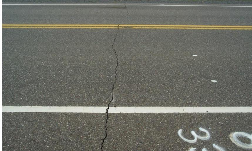
**Figure 100.15** – Transverse Thermal Crack
