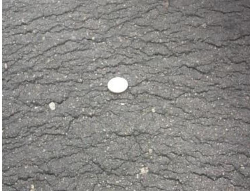
Figure 600.22 – Checking of the mat
