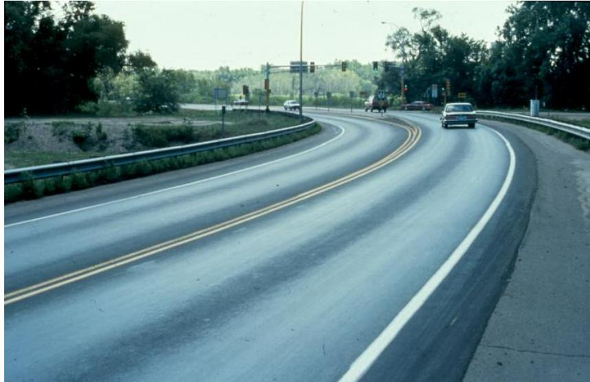
Figure 600.11 – Pavement Flushing
