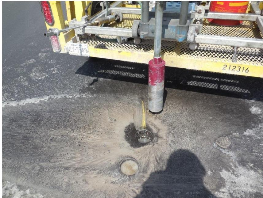
Figure 500.26 – Core Drill
