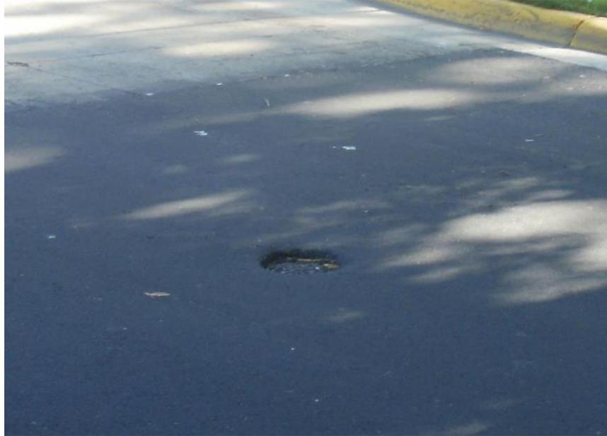
**Figure 500.30** – Water valve box that has been adjusted too low.
