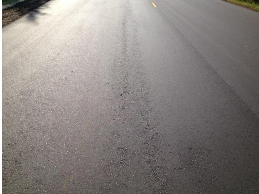
**Figure 600.9** – Moderate segregation of the pavement
