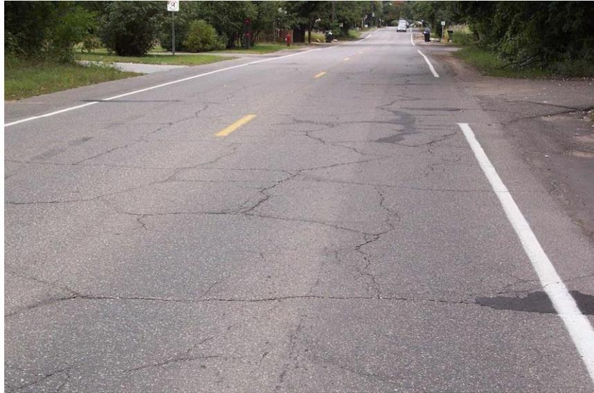
**Figure 100.16** – Block Cracking
