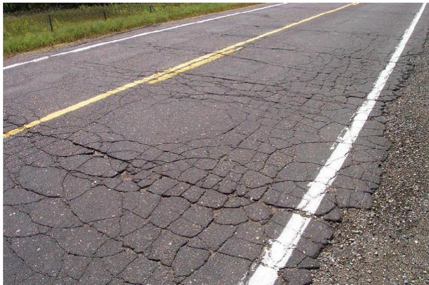
**Figure 100.17** – Severe Fatigue Cracking
