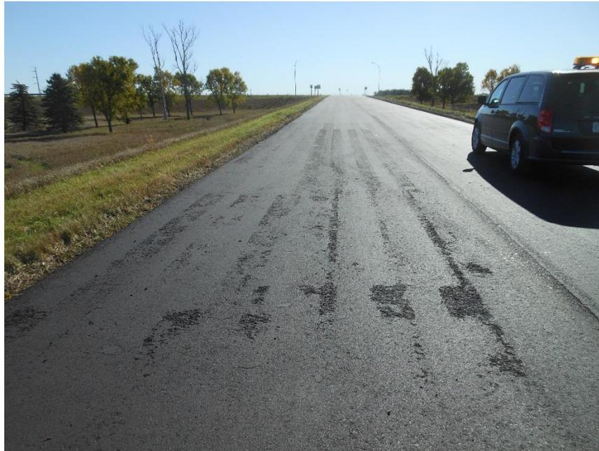
**Figure 500.32** – Unacceptable mixture pickup from pneumatic tired roller
