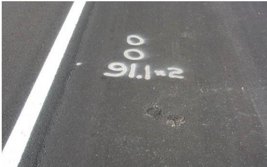
**Figure 700.12** – Core locations marked on the roadway. Note that the cores were not taken in the marked locations. These cores must be recored at the proper locations.
