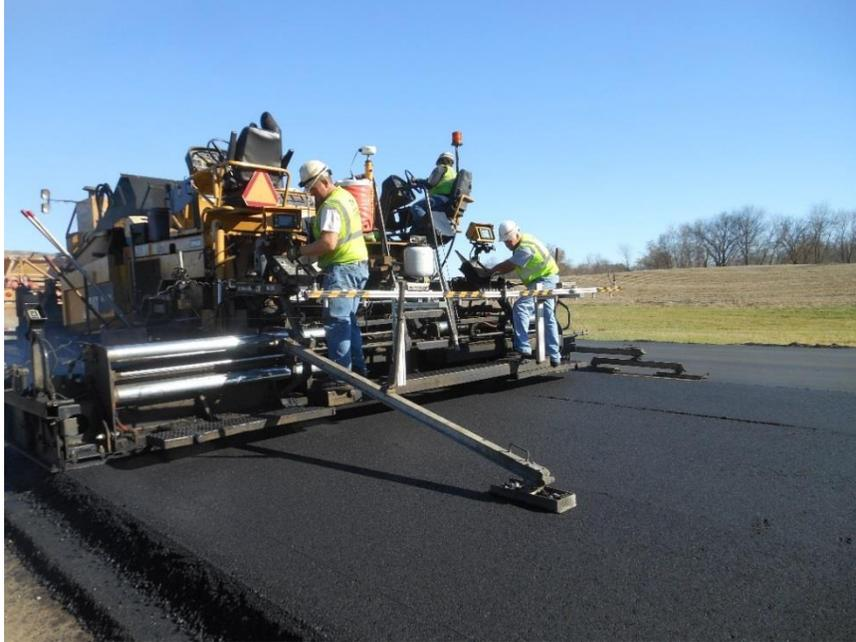
**Figure 600.20** – Lines in the mat from incorrectly adjusted screed extensions.
