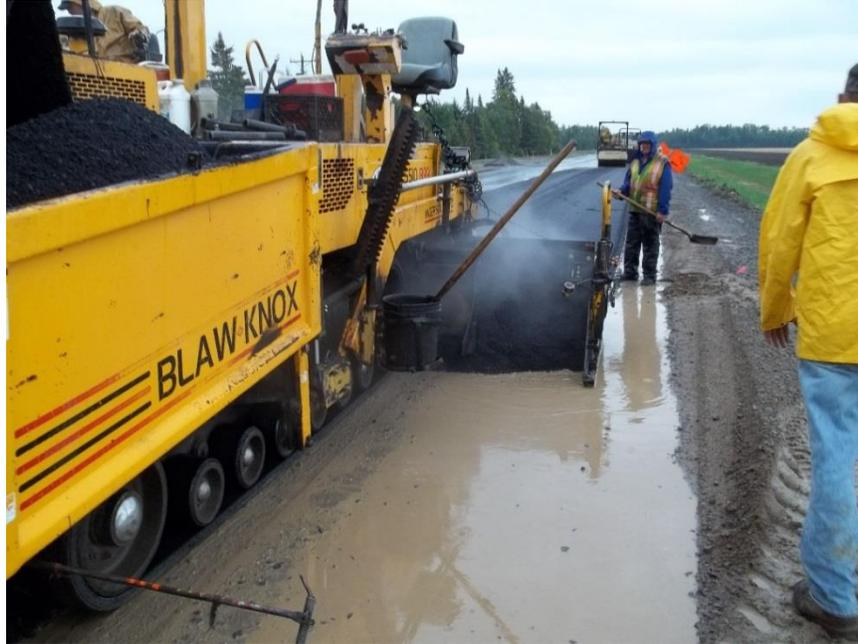
**Figure 600.34** – Paving in the rain. When the paver creates a wake through the water, it is well past time to halt production. The situation pictured above should never be allowed to occur.
